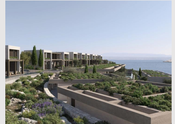
JW MARRIOTT CRETE RESORT & SPA In progress 160 rooms | Investment Value 80M
