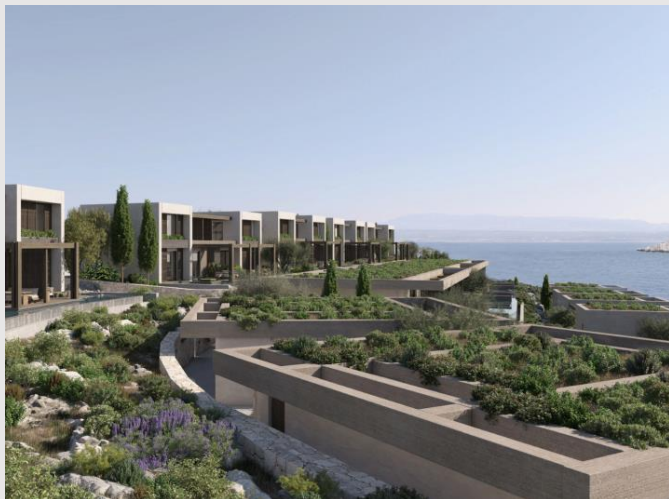
JW MARRIOTT CRETE RESORT & SPA In progress 160 rooms | Investment Value: 100M
